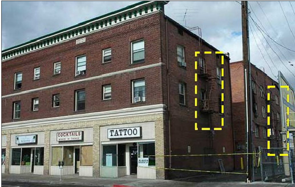
Figure 6. Rear Fire Escapes.
