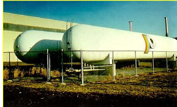
**Ultrahigh-pressure** containers such as tube tanks, pipelines, or cylinders are not common and contain mostly gases and a few liquids. They are usually aboveground and horizontal.
