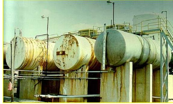
**High-pressure** containers such as propane and other compressed gas cylinders can be found as spheres or cylinders above or belowground. A common example is medical oxygen cylinders. High-pressure containers normally hold gases, liquids, or powders.
